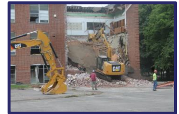
DEMOLITION OF EXISTING BUILDINGS
