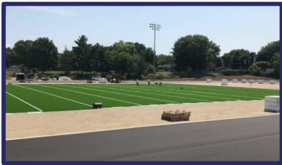
NEW STADIUM TURF / EARLY SITE
